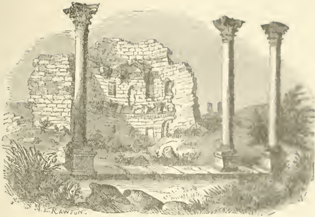
Part of the principal street, Gerash.
